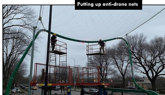
Putting up anti-drone nets
